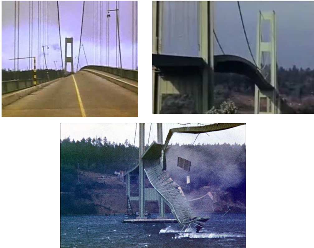
Figura 20 – Colapso da Tacoma Narrows Bridge
